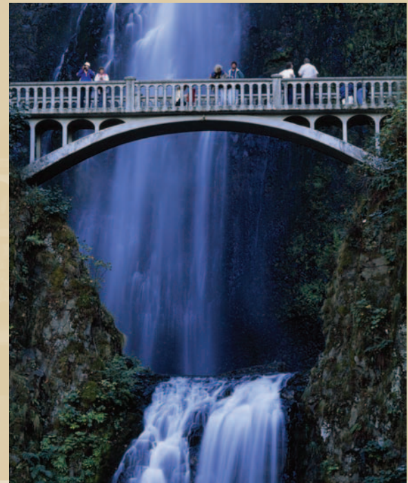
Columbia River Gorge, Oregon, bridge at Multnomah Falls © Rich Reich/National Geographic Image Collection
