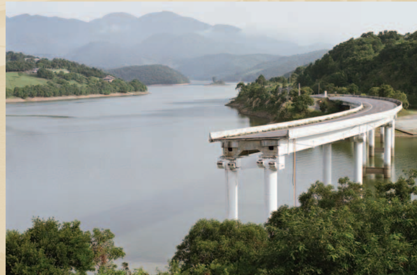
Brazil, Sao Paulo, Curitiba motorway under construction © Jens Lucking/Stone/Getty Images
