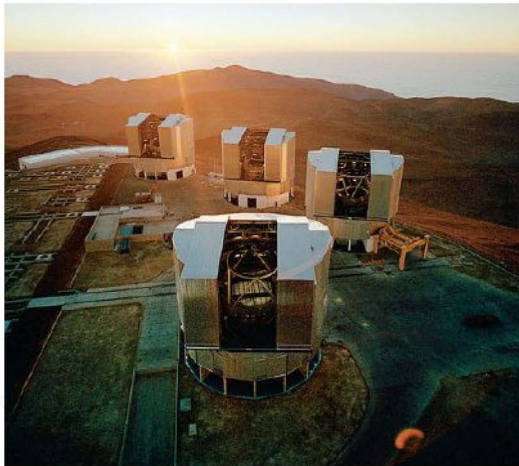
▲ FIGURE 5.10 VLT Observatory Located at the Paranal Observatory in Atacama, Chile, the European Southern Observatory's Very Large Telescope (VLT) is the world's largest optical telescope. It comprises four 8.2-m reflecting telescopes, which can be used in tandem to create the effective area of a single 16-m mirror. ( ESO )
